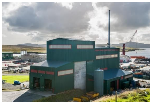
Figure 3-4: Lerwick energy recovery plant [28]
