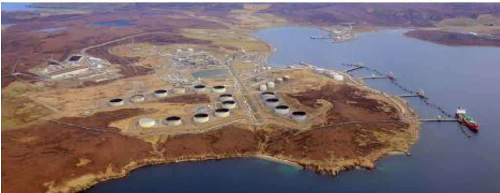
Figure 5-2: Sullom Voe Oil Terminal, Shetland Islands [27]
